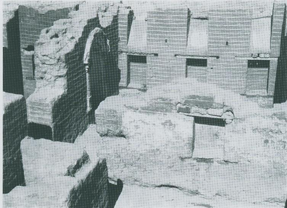
86 A private house at Karanis. A view into a substantial mud-brick house of the Roman period, showing the interior walls with unusually regular brick courses. The niches beneath the windows are surmounted by wooden lintels and will have served as storage cupboards. The wall at the left contains a shrine niche which has fluted columns, capitals decorated with scrolls and a shell-shaped top.
