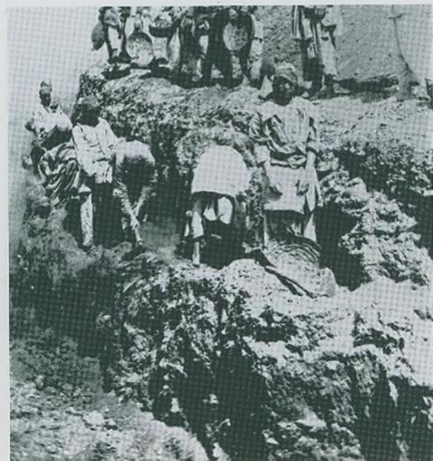
96 Excavations at Oxyrhynchus, c. 1900. The rubbish tips of ancient towns were plundered for fertiliser ( sebaki ) by the modern inhabitants and the resulting casual finds of papyri eventually led to systematic excavation of such dumps at the turn of the century. The town of Oxyrhynchus has proved by far the most productive of such sites.
