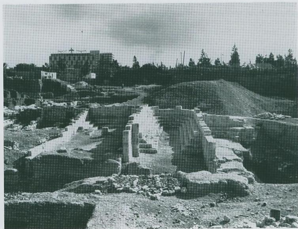
141 Alexandria (Kom-el-Dik), a school. This unique building which lies close to the theatre and the baths consists of three elements. In the centre is a main lecture hall, with the lecturer's seat at the centre of the short range at the top; the rooms on either side are smaller and may be subsidiary classrooms or preparation rooms – the one on the left is square-ended, the one on the right horseshoe-shaped.
